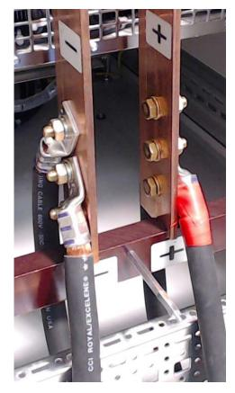
Always use wire lugs to connect the output cables to the bus bars. The above figures show the proper placement of the hardware against the bus bars.
