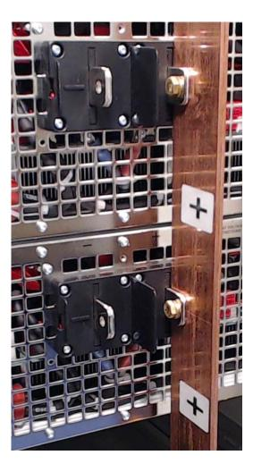
3. Continue with the negative bus bar. Place the negative bus bar on the bottom support bracket. Position the bus bar on the left side of the negative output terminals. Repeat step 2 for the negative bus bar.
